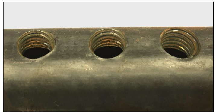
FIGURE 6: Unacceptable Rust in Coupler Threads
