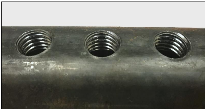
FIGURE 5: Clean Acceptable Coupler
