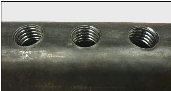
FIGURE 5: Clean Acceptable Coupler
