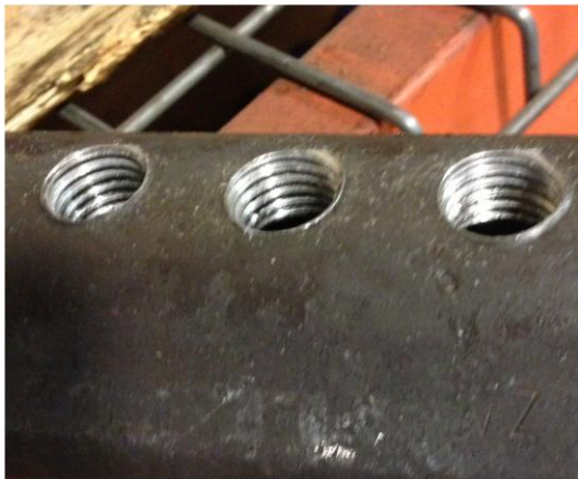
Figure 6. Clean Acceptable Coupler
