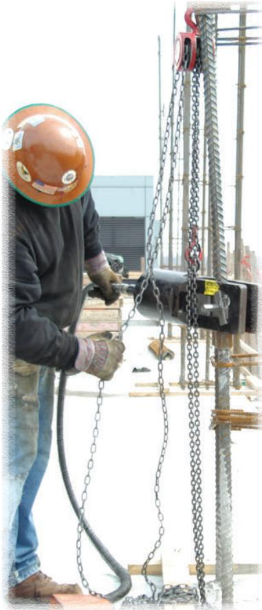
**BarGrip XL cold-swaged coupling sleeves** consist of seamless steel sleeves that slip over the ends of reinforcing bars. They are swaged onto the reinforcing bar profile to produce mechanical interlock.
