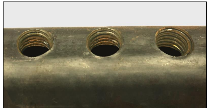
FIGURE 6: Unacceptable Rust in Coupler Threads
