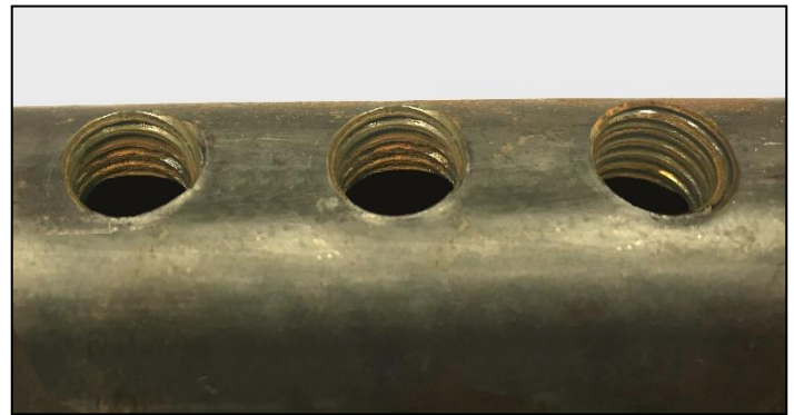
FIGURE 6: Unacceptable Rust in Coupler Threads
