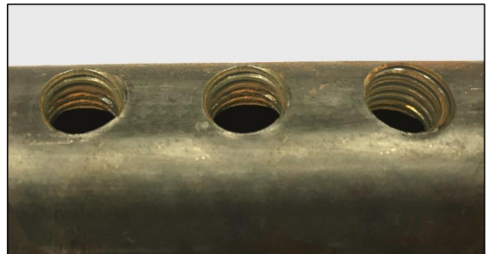
FIGURE 6: Unacceptable Rust in Coupler Threads
